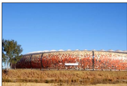
Soccer City Stadium i Johannesburg.
